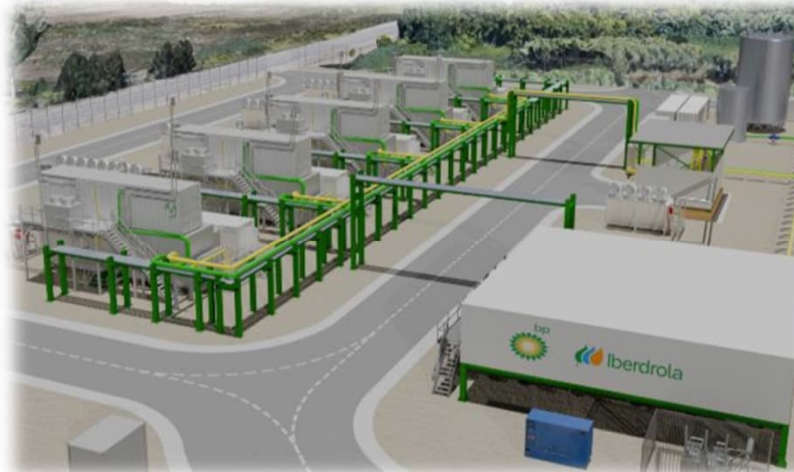
25 MW mock-up plant – 5 modules of 5 MW
