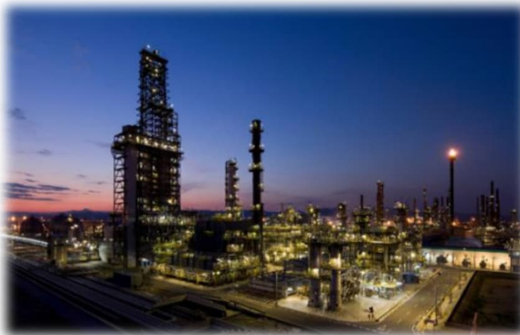
bp's refinery in Serrallo Industrial Park, Castellón
